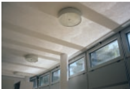
Fig. 1: Example of an effect of light-deflecting glazing, which cannot be calculated with existing simulation tools.
