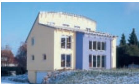
Free-standing passive house in Hohenstein.
