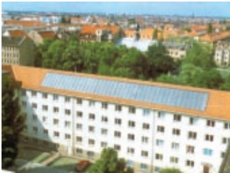
Fig. 1: System with a large collector area on a multi-storey building, from the "Solarthermie 2000" programme.
