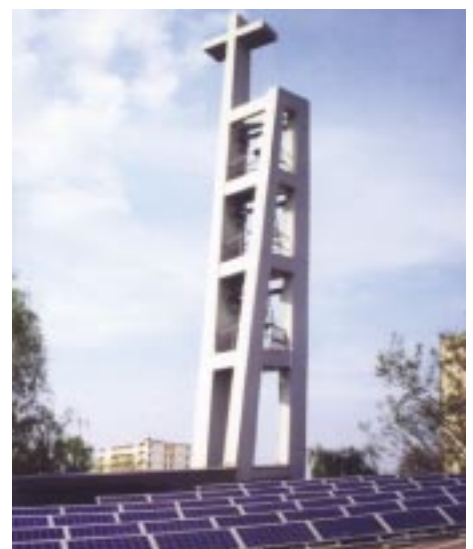
Fig. 3: The system belonging to the Catholic Students' Congregation in Berlin has a specific annual yield of 680 kWh/kW p , which is considerably lower than the average.
