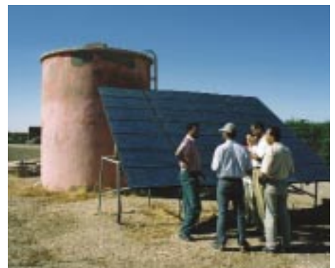
Fig. 1: PV-powered water supply in Efert, Morocco, with an integrated disinfection plant. In future, a miniature electricity grid based on photovoltaics should also be installed in the village.
