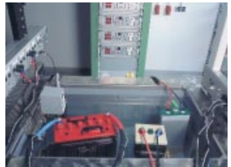
Fig. 1: We have a total of more than 50 battery testing circuits for short-term and long-term electrical characterisation, with current ranges between 20 mA and 300 A and voltages between 1 V and 500 V. Three water baths and two temperature-controlled cabinets are available to keep the battery temperature at the required value.
