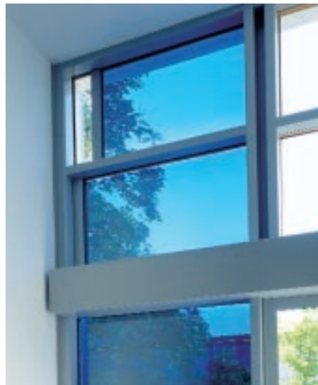
Fig. 1: Test façade with coloured and bleached switchable (gasochromic) windows at Fraunhofer ISE.
