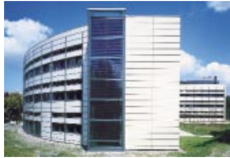
Fig. 1: A 2.4 kW p photovoltaic generator is integrated into the end façade of the access tract.
