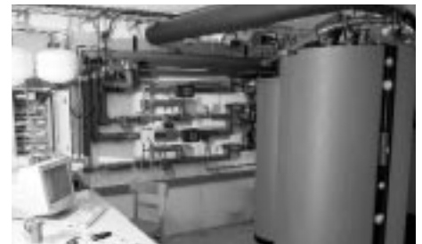
Fig. 2: Sorption storage unit in the Freiburg Solar House. The photo shows two containers filled with sorption agent and a water tank, which also contains the evaporator and condenser.
