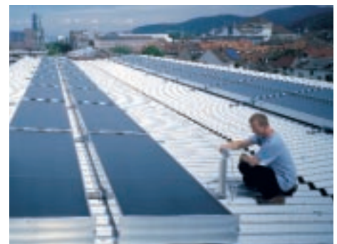
Fig. 2: Solar air collector system on the roof of the Chamber of Commerce for the southern Upper Rhine region.
