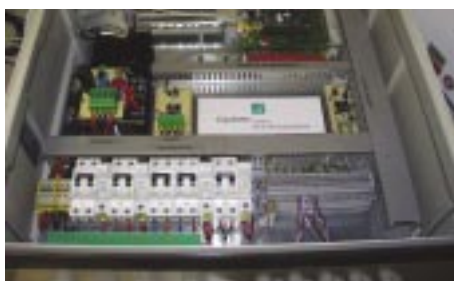
Fig. 2: Electronics of the energy management system to control hybrid systems.
